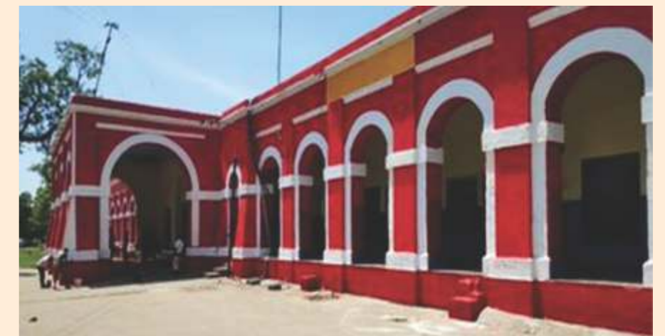
Rajmahal Station after renovation
