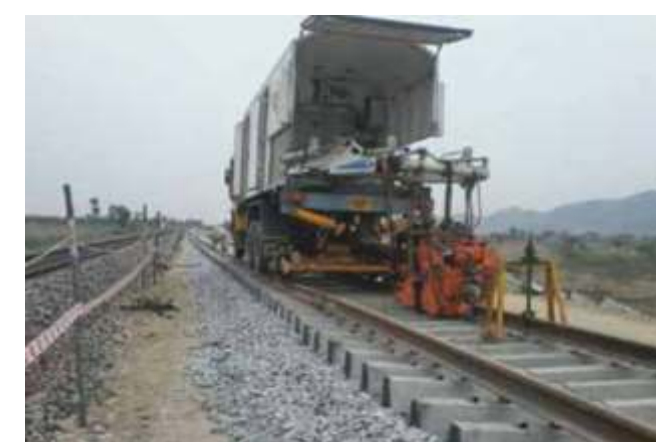
Flash Butt Welding
